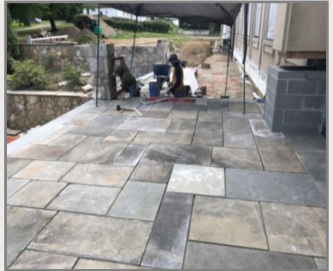
New sidewalks and stonework
