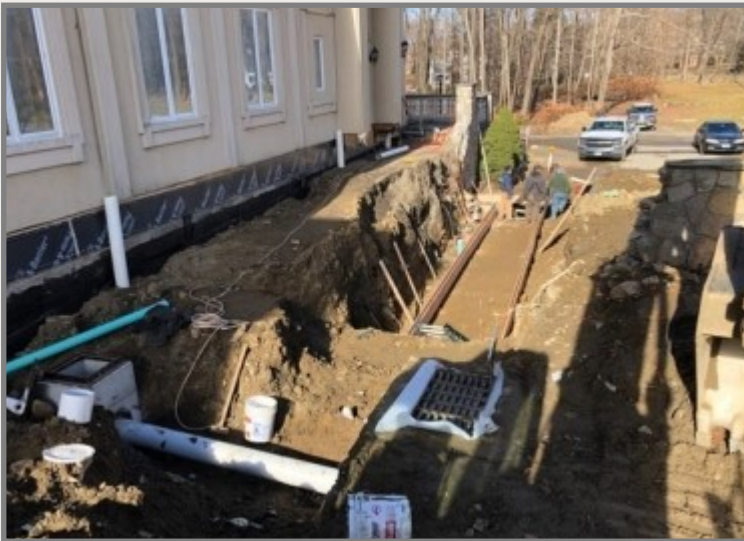
Drainage installation and grading
