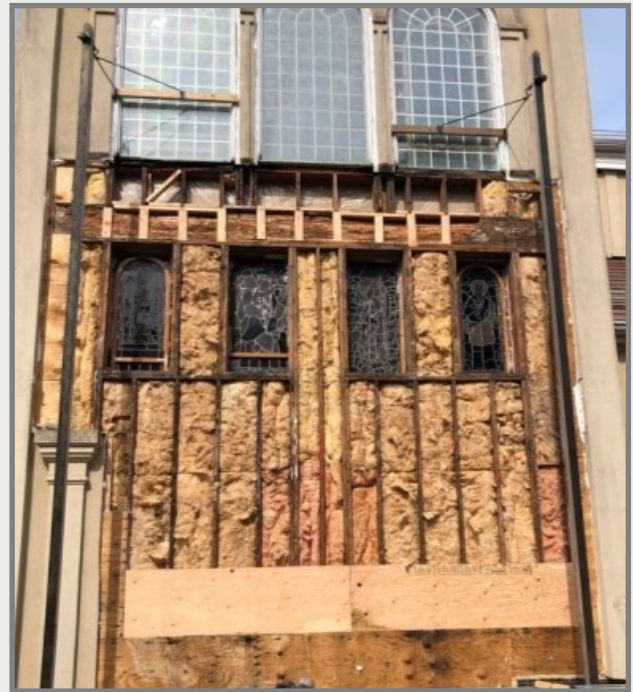
Extensive façade repair
