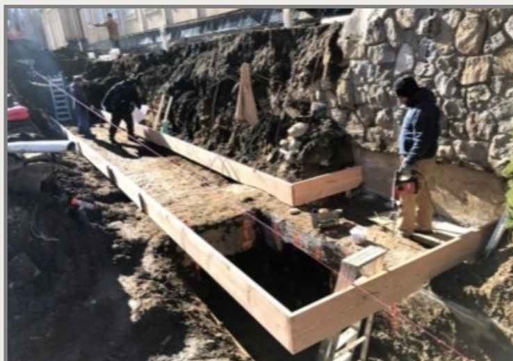
Reconstruction of retaining wall and stonework
